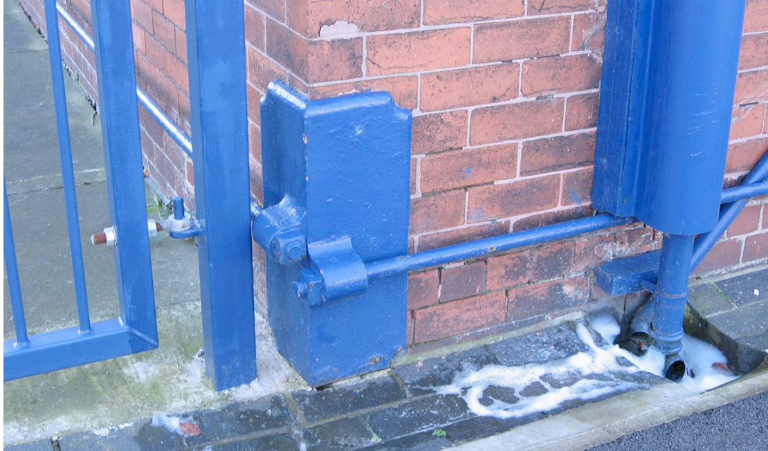
Sutton Manor Blue brackets supporting local school against subsidence, St.Helens, 2007
